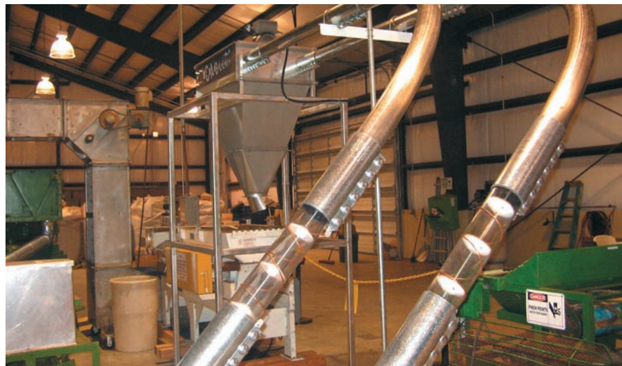
Close-up of Inspection Tube shows tea moving.
