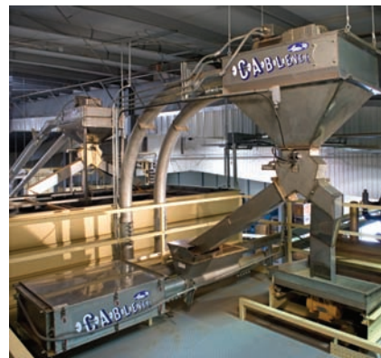
Almonds are transferred from one tubular drag conveyor (top) to another (bottom).
